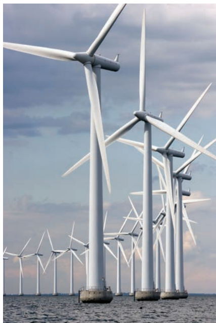
FIGURE 39.9 Offshore wind parks. Capacity factors at near-offshore locations like this one in Denmark are generally higher than on land. (Max Muelie/Alamy)
