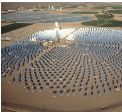
FIGURE 39.5 A concentrating solar thermal power plant. Mirrors and reflectors concentrate the energy of the Sun onto a “power tower,” which uses the sunlight to heat water and make steam for electricity generation. (Lowell Georgia/Science Source)
