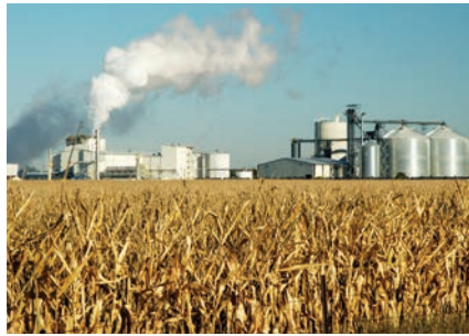
FIGURE SA6.1 An ethanol-producing factory. Ethanol-producing factories, such as this one in South Dakota, convert corn into ethanol to produce a fuel that can be mixed with gasoline to power automobiles. (Jim Parkin/Alamy)
