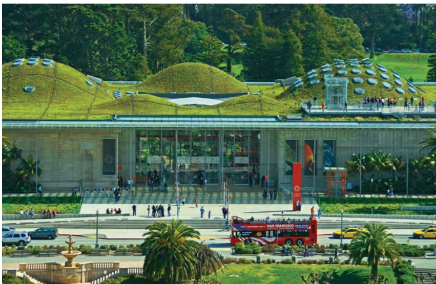
FIGURE 37.4 The California Academy of Sciences. The sustainable design of this San Francisco research institution maximizes the use of natural light and ventilation. The building generates much of its own electricity with solar panels on its roof and captures water in its rooftop garden. (Nancy Hoyt Belcher/Alamy)
