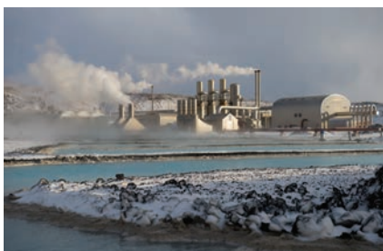
A geothermal energy power plant in Iceland. This thermal power station in west Iceland uses geothermal energy from Earth rather than a fossil fuel to produce electricity and hot water. (Felipe Cui-Paoluzo/Getty Images)
